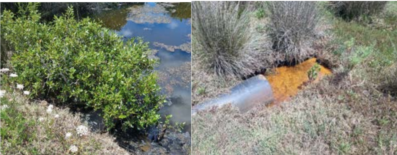
Figure 2-2 Eastern culvert (Upstream and downstream)
