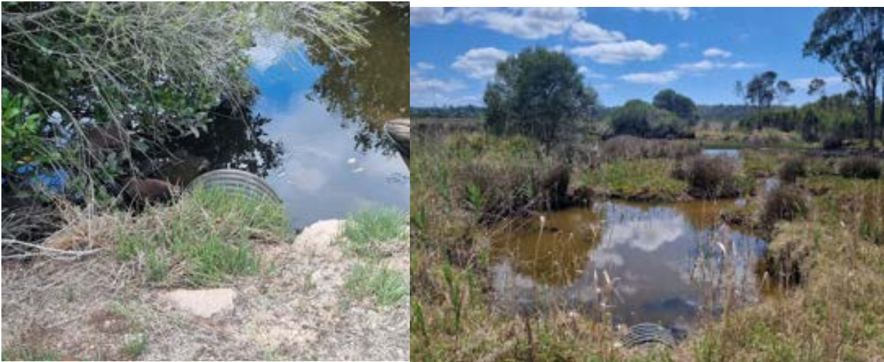
Figure 2-1 Southern culvert (Upstream and downstream)
