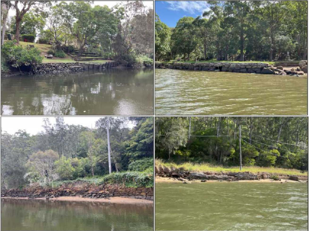
Plate 16 Examples of partially effective bank protection works in the Georges River estuary, clockwise from top left: failing timber wall in Prospect Creek Reach 1093; failing rock wall adjacent to public park area in mid Georges River Reach 416; failing gabions and concrete wall in the lower Georges River Reach 463; and failing rock wall in the Woronora River Reach 636.
