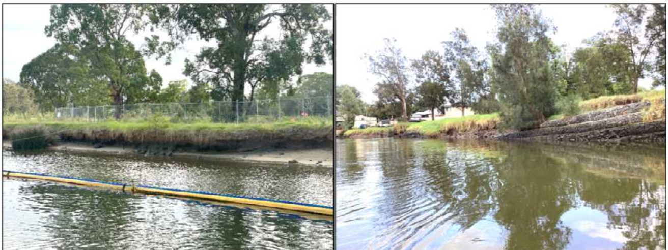
Plate 1 From left to right: boat wave wash erosion is common in the Fluvial Dominated process zone particularly around Milpera (upper Georges River Reach 250); bank toe scour and slumping and typical processes occurring in the Fluvial Dominated process zone.
