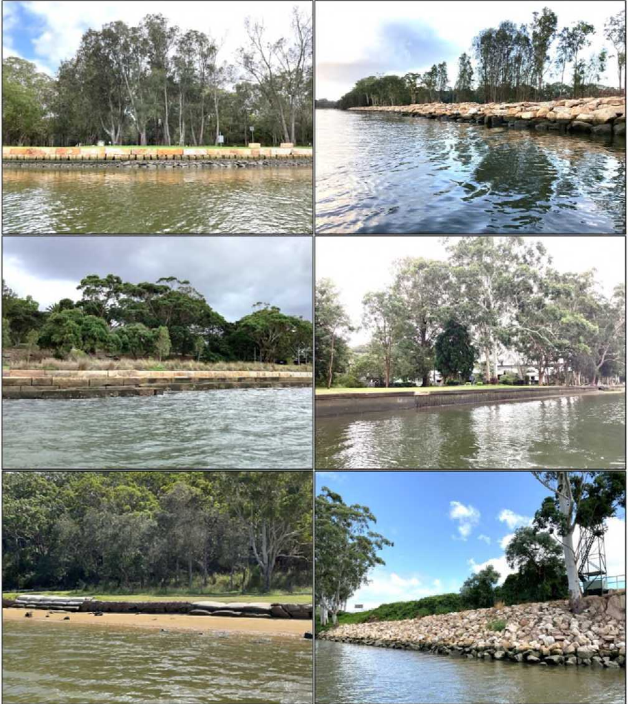
Plate 15 Examples of effective bank protection works in the Georges River estuary, clockwise from top left: sandstone block wall and rock armour toe on the mid Georges River Reach 291; upper Georges River Reach 162; geotextile sandbags used in a public access location on the mid Georges River at Reach 426; and rocky foreshore habitat restoration at Carss Park Reach 989.
